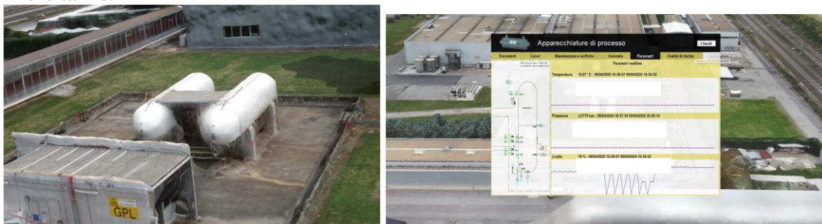
Figure B.5.3 Details from the SECURDOMINO software for DEMO2: a) Detailed view of the LPG tanks; b) snapshot of real-time data interface.
